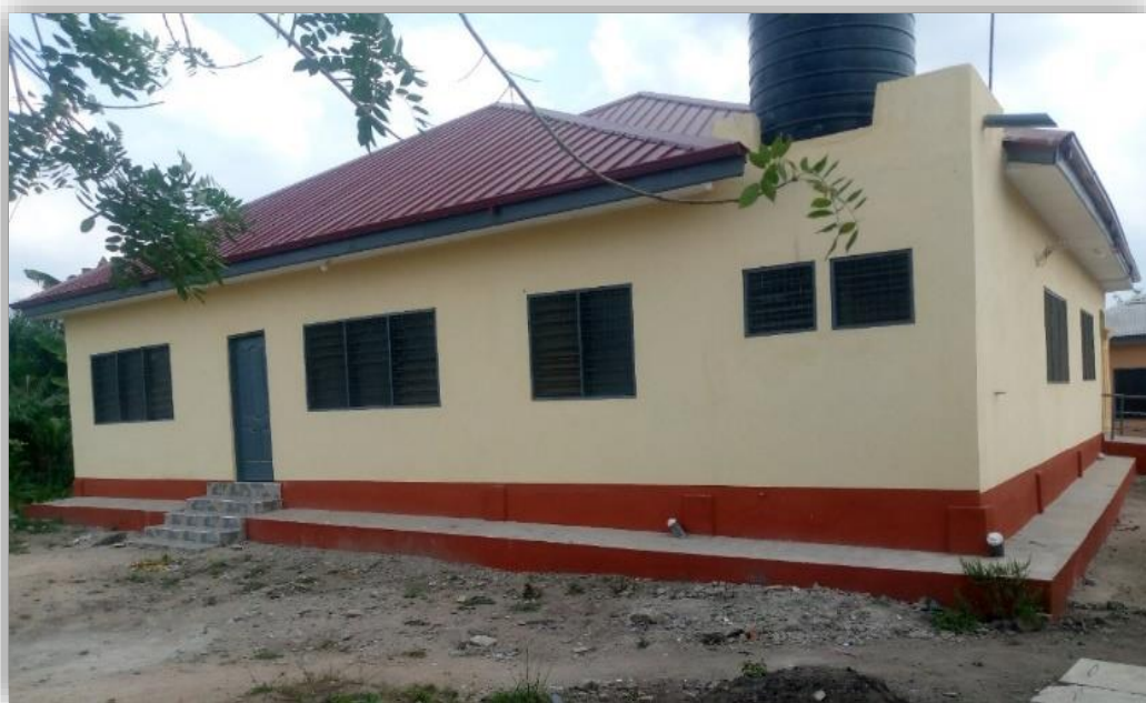
Figure 2.18: Maternity ward at the Kpetoe Health Centre
